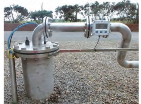
Modern borehole construction.
